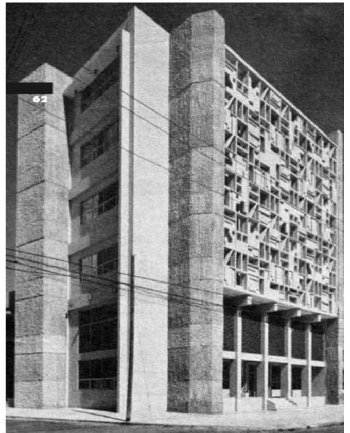
3. Wilson Chong, Henriques Building
