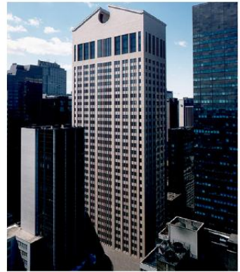
4) AT&T Building, Philip Johnson
